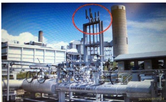
Vent pipe for pilot valve
